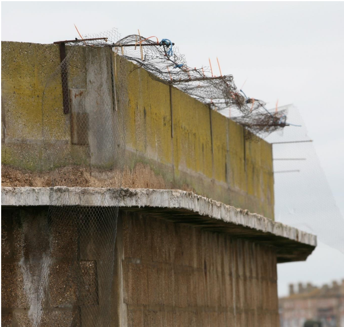
Photo 3.4.5. The artificial ledge in 2021, showing the upper ledge and wire mesh put above, possibly intended to exclude herring gulls from landing on the ledge
